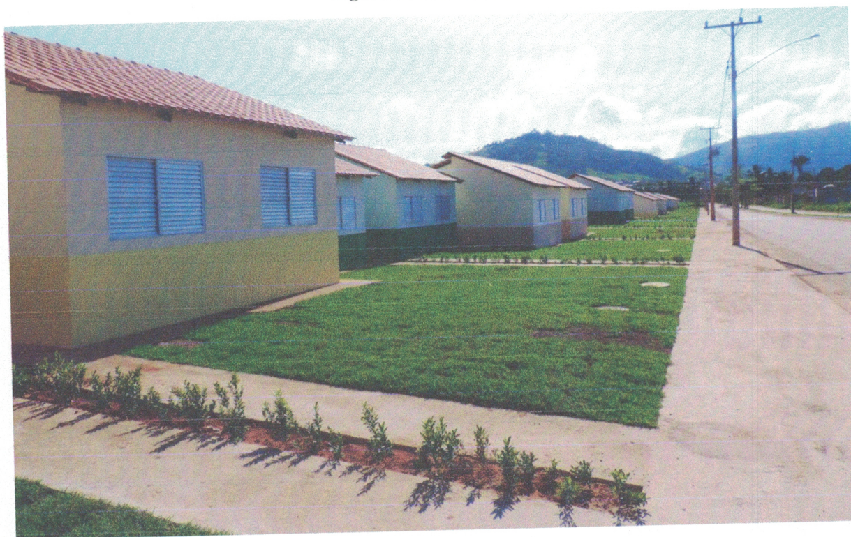
Figura 5. Residencial Vale do Sol I.
